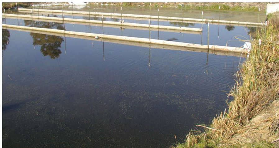
FIG. 4. Pilot-scale open-water wetland cell located in Discovery Bay, CA. The cell is about 20 cm deep, 400 m 2 , and has a hydraulic residence time of about 3 days.
