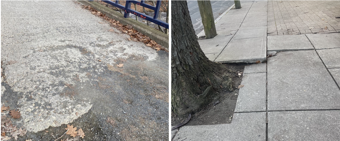
Figure 10: Examples of weathering that is problematic for accessibility. Left: Potholes on the bridge to the Smith athletic fields. Right: Uneven sidewalk outside of the Smith bookstore.
